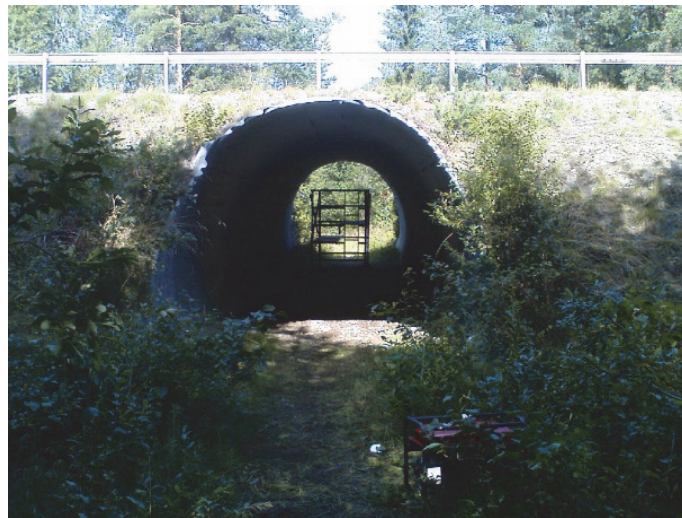
Figure 1. Flexible culvert in northern Sweden built 1966. Measurements under live load were performed in 2012 recording crown deflections and steel strains.
