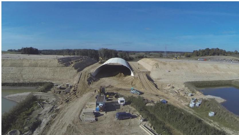
Figure 4. Structure during backfilling
