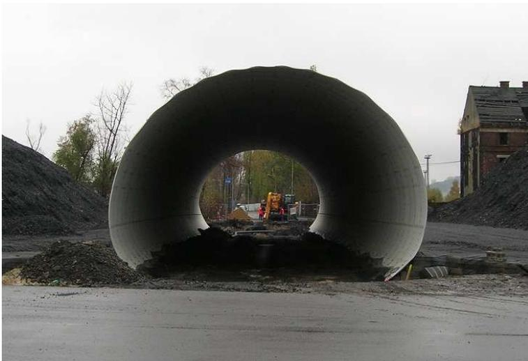
Fig. 3. Structure after assembly, before backfilling
