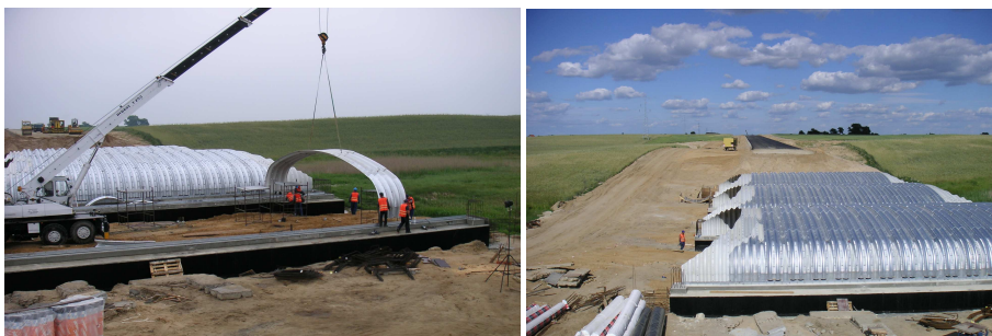
Figure 1 Deep corrugated steel box grade separation under construction
