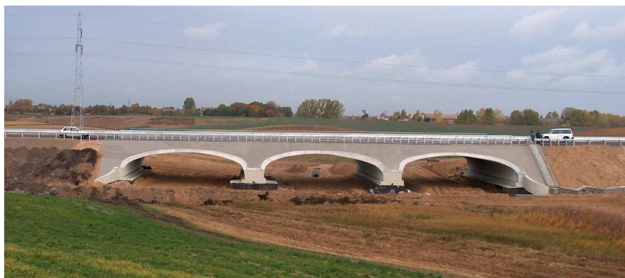
Figure 2 Ready bridge directly after completion
