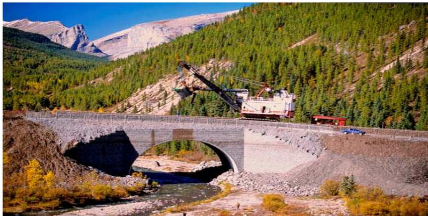
Fig. 1. Soil-steel bridge in White Horse Creek [1]
