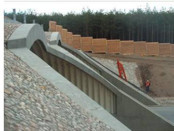
Figure 14. Side view of concrete collars for arch structures
