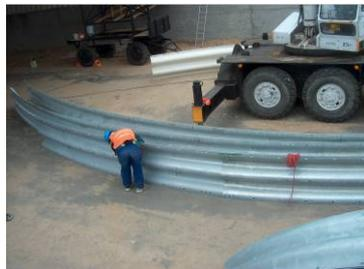
Figure 8. Pre-assembly of top plates of arch on the ground
