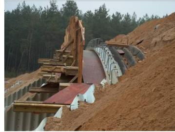
Figure 13. Construction of formwork for concrete collars for arch structures
