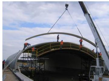
Figure 9. Assembly of pre-assembled top plates of arch
