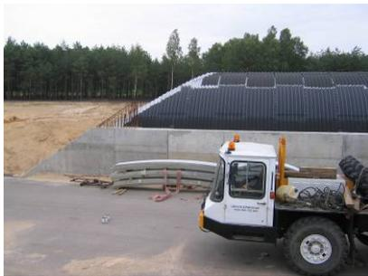
Figure 6. Structure painted with bituminous coating from the backfill side
