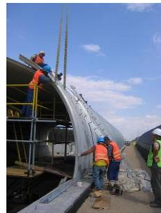
Figure 7. Assembly of side plates of arch to the base channel
