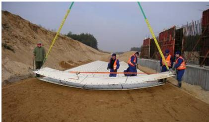
Figure 2. Assembly of bottom plates of close shaped structure on prepared bedding
