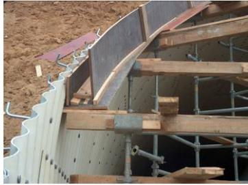
Figure 12. Construction of formwork for concrete collars for closed structures
