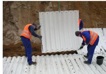
Figure 3. Assembly of side plates of closed structure
