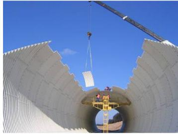
Figure 4. Assembly of top plates with using of plate-by-plate method
