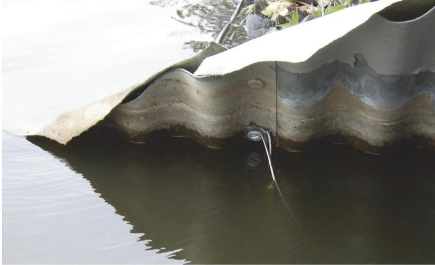
Figure 5. Cathodic protection anodes attached to a culvert
