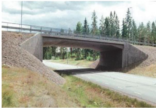
Figure 1. A concrete slab frame bridge [18]
