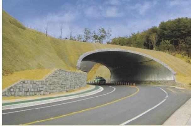
Figure 2. A steel soil composite bridge [19]
