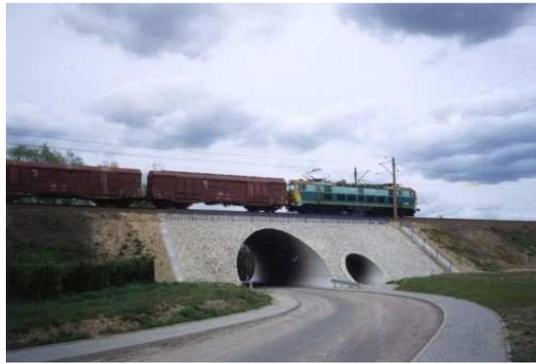
Fig. 1: Two corrugated flexible culverts beside each other used to carry a two track railway line over a road and a foot-path in Poznan, Poland.
