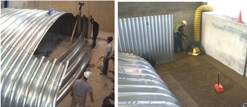
a. Erecting the 10m span box culvert    b. Culvert being backfilled with GW-SW soil
