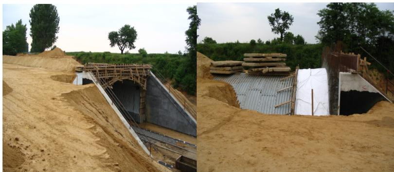
Figure 4. Ballasting with use of soil and concrete panels
