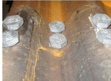
(b) the modified 4 bolt – non crack
